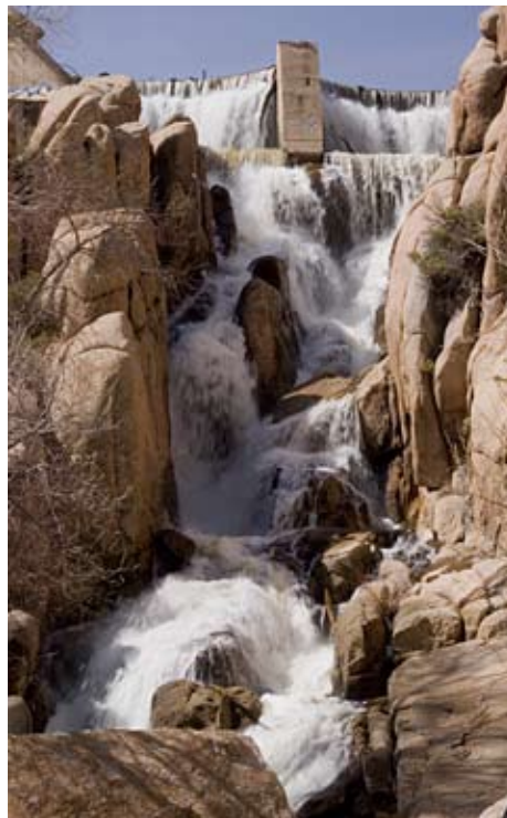
Watson Lake spillway as it enters Granite Creek Photo: Alan Smith
